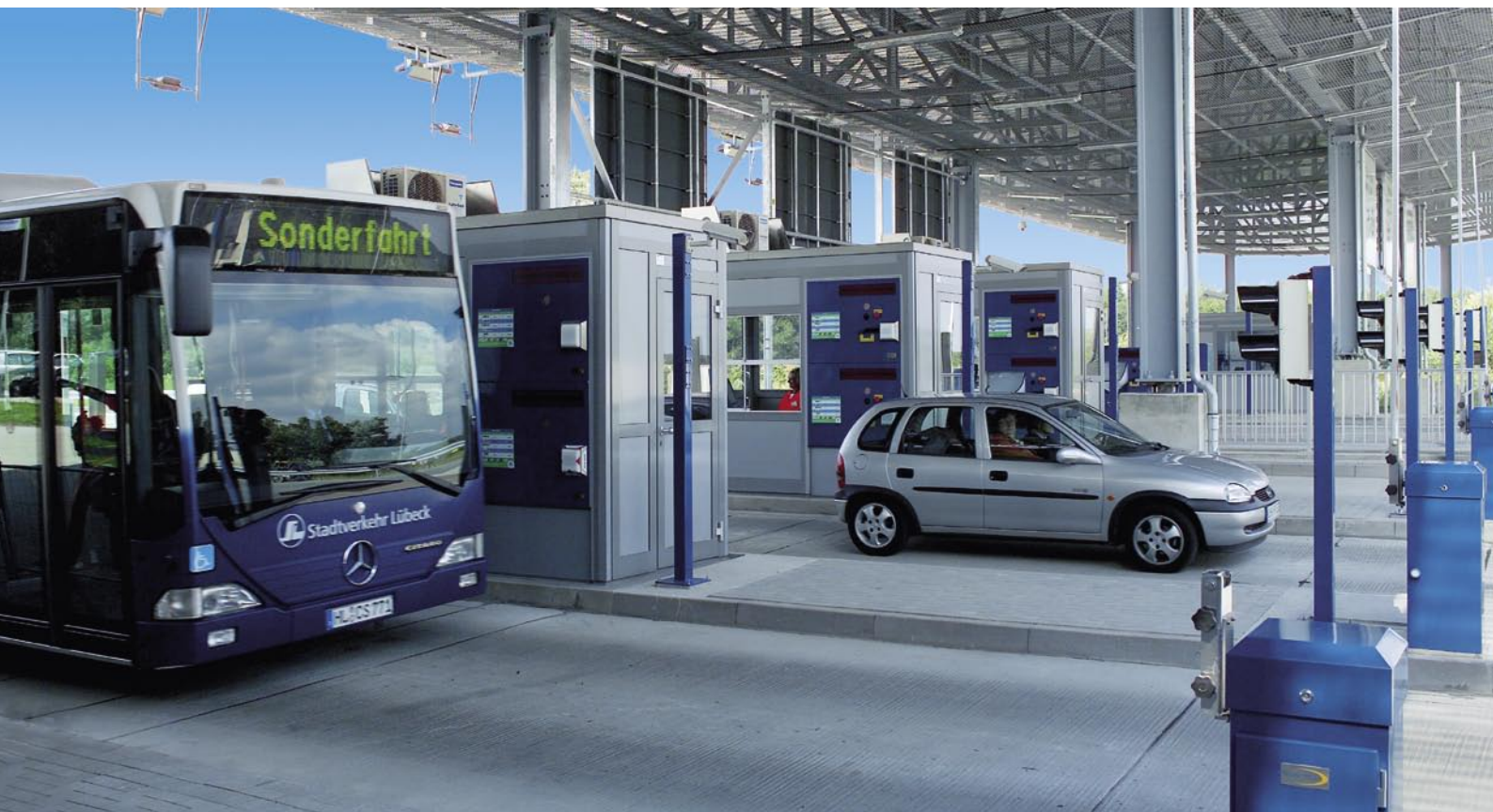
Herren Tunnel Lübeck, one of the first toll roads in Germany, opened in August 2005. The project is an outstanding example of efficient public-private partnership.
