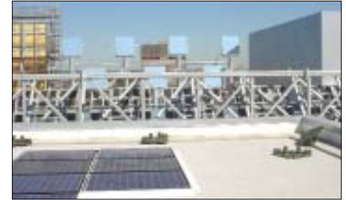
Heliostats and powered mirrors track sunlight and reflect it into the atrium at Genzyme Center, Boston, Mass.
